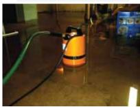
The Surface Level Switch is used to automate a utility/floor sucking pump. Set the Surface Level Switch on the floor and plug the power cord from the pump into the piggyback plug on the switch. Plug the piggyback plug into a standard 120 VAC wall outlet (the unit will also work on GFI outlets).
